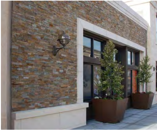
Pre cast concrete with stone cladding creates a refined storefront.
