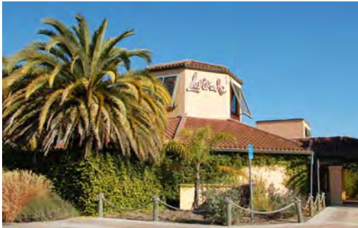
Stucco walls with terra cotta roofs are appropriate for Mediterranean style buildings.
