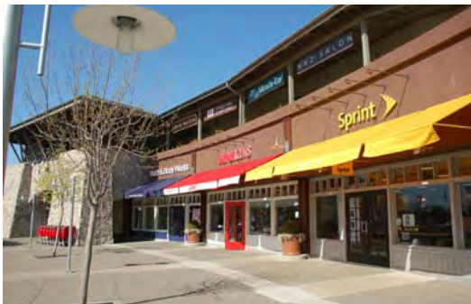
Awnings help scale the building to the pedestrian.
