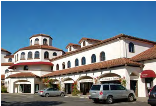
Hipped roofs with eave overhangs.
