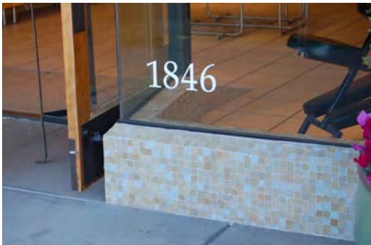
Glass tile bulkhead gives a fresh, modern look.
