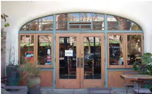
The integration of doors, storefront windows and transom windows provides a striking storefront.
