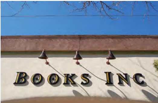
Wall mounted signage with gooseneck lighting.
