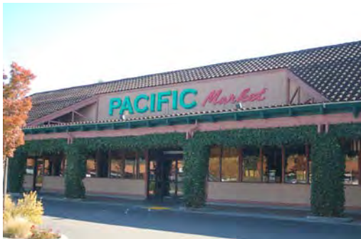
Wall mounted exterior lit signage.
