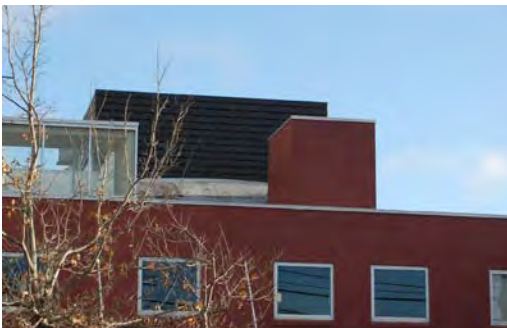
Roof mounted equipment screening is integrated with the building volumes.
