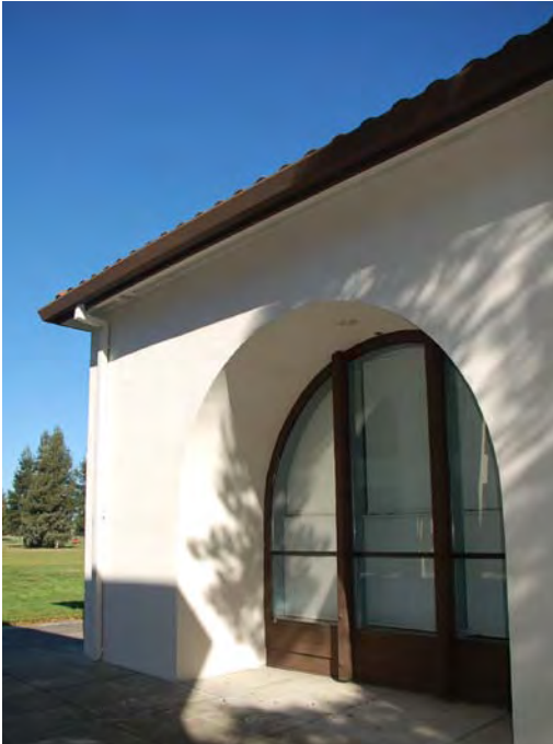
Deeply recessed windows create a dramatic effect and cast shadows on the facade.
