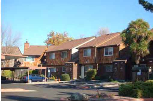
Two story attached multi-family housing.
