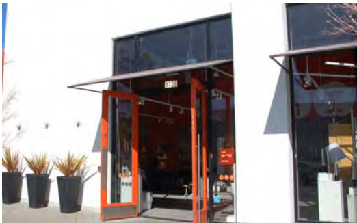
Transom windows accent storefront entry.
