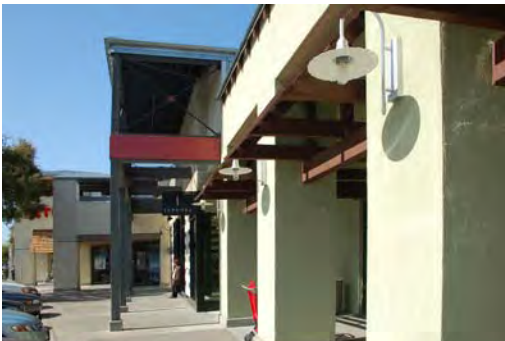
Wall mounted sconces at arcade.
