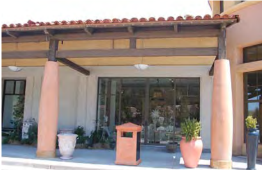
Display windows are consistent with the shape of the arcade opening.
