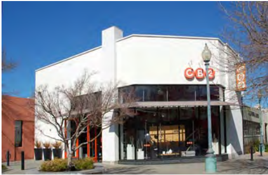
Awnings between the storefront and transom windows provide storefront hierarchy and shading.
