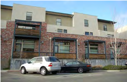
Brick at the ground floor adds nice contrast to the smooth stucco above.
